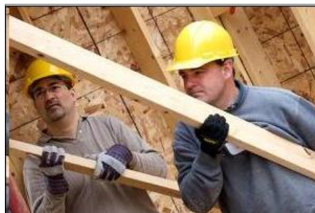
Volunteers from EMC help raise the roof in Ashburnham
